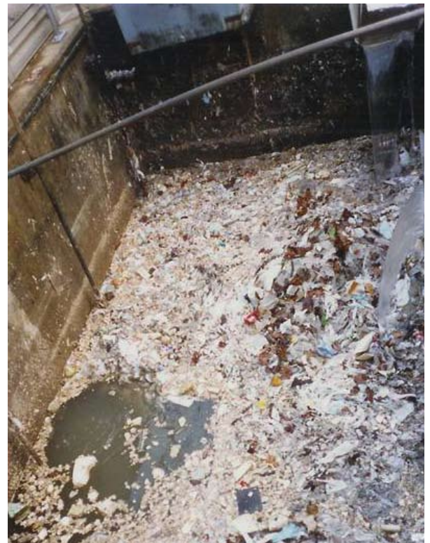
Accumulation of material floating on surface of sump
